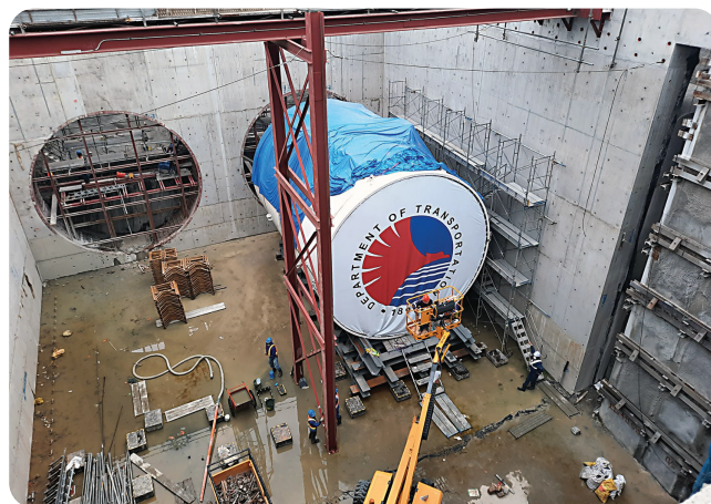
The Metro Manila Subway Project under construction.
